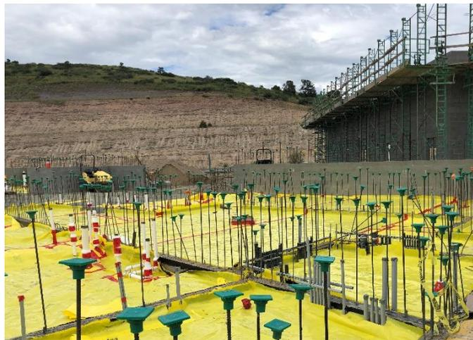
FIGURE 1 – VAPOR BARRIER BEING PLACED IN AREA B PRIOR TO SLAB ON GRADE PLACEMENT
