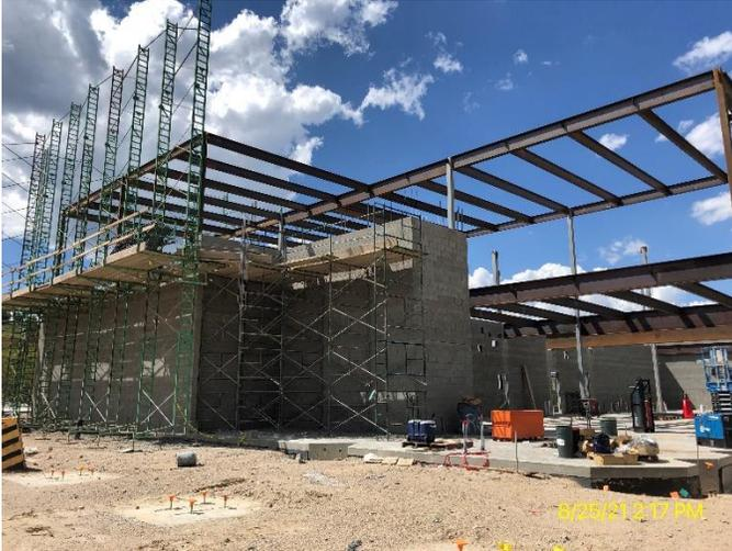
FIGURE 3– STRUCTURAL STEEL PLACEMENT IN THE FUTURE COURTS.
