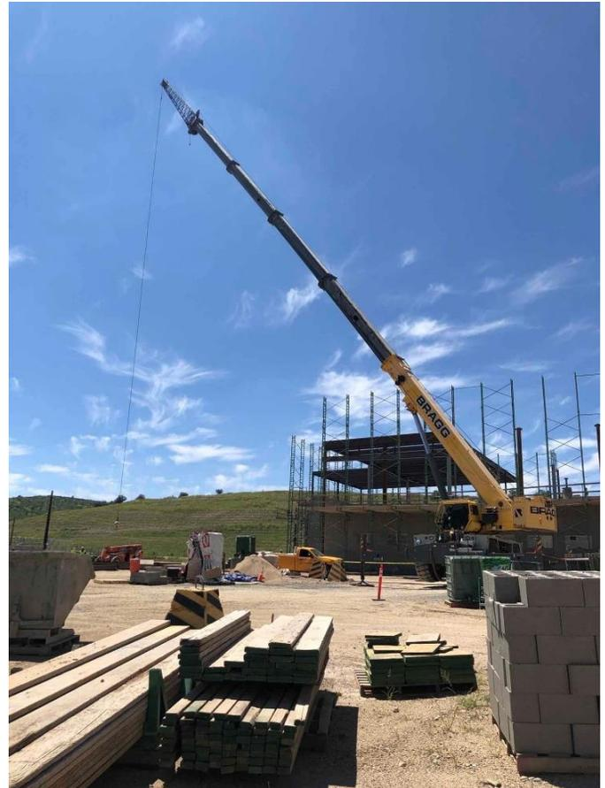
FIGURE 2 – CRANE HAS BEEN DELIVERED TO THE SITE. IT WILL BE USED FOR THE INSTALLATION OF STRUCTURAL STEEL.
